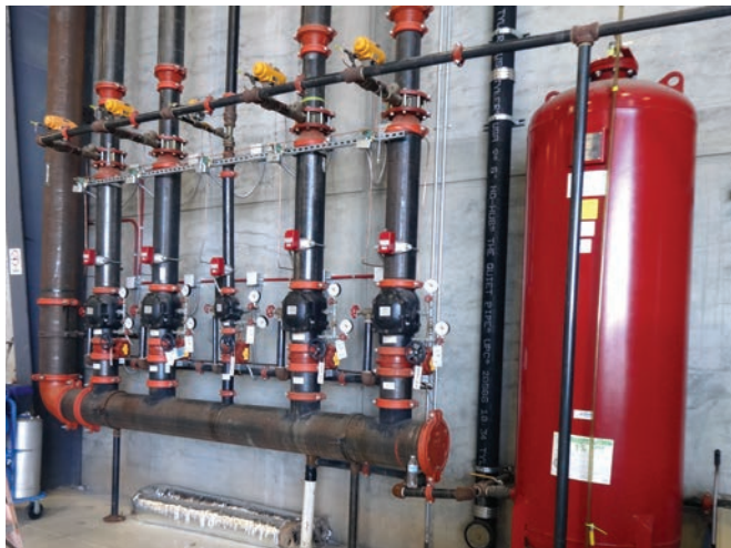
Risers with bladder tank.
