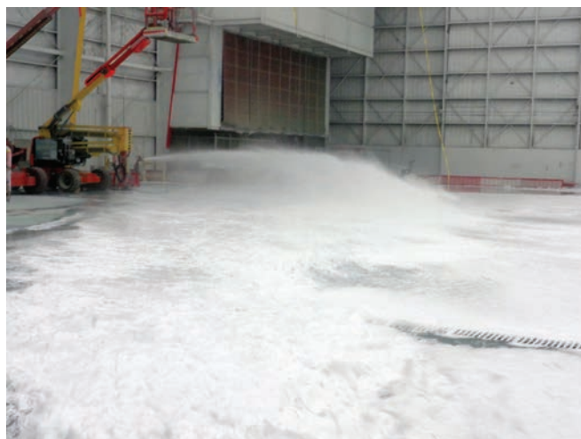
Oscillating monitor foam discharge.
