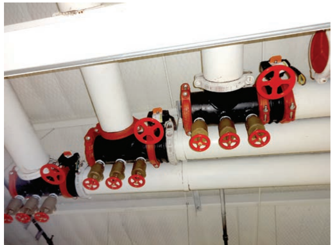
Riser test connections.
