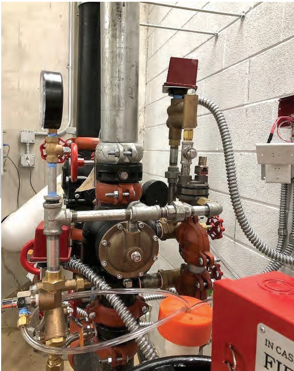
Installed Victaulic Series 769N Non-interlock Preacton Trim Configuration (Image credit: Victaulic)
