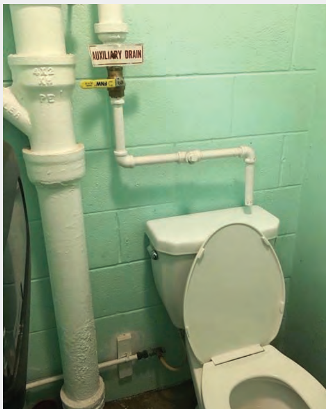
Photo taken a couple of years ago by Henry Fontana, Orange, CA Henry@HenryFontana.com
